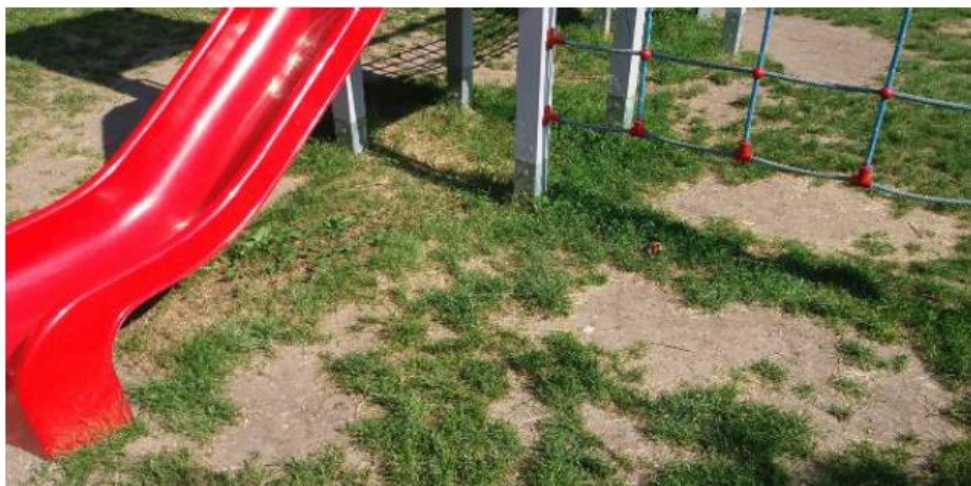
Photograph 14: An example of unsafe surfacing in a playground in the Czech Republic
