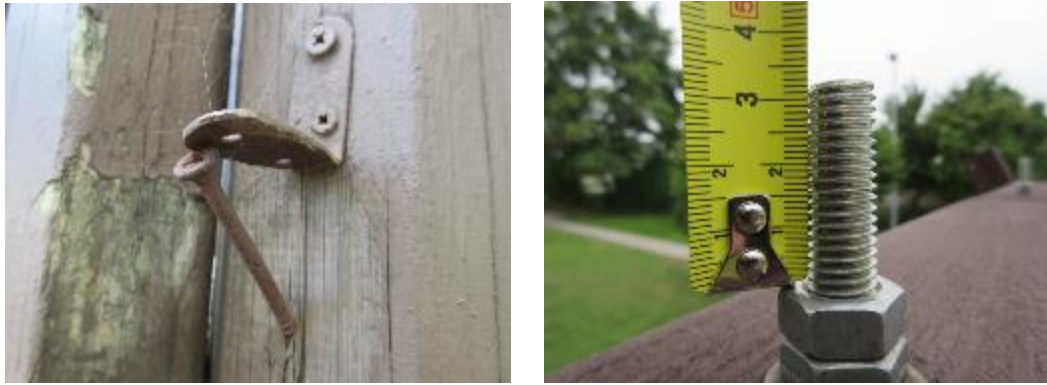
Photograph 8: Projections on items of equipment in Latvia
