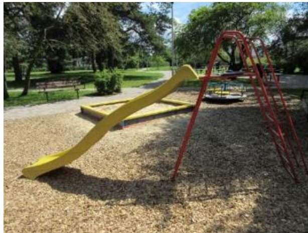
Photograph 9: A slide in a Latvian playground where there is a failure to protect from a fall
