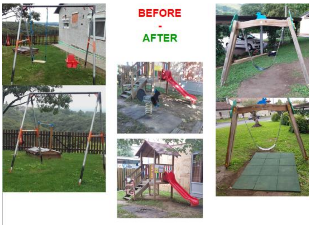
Photograph 19 Examples of post-inspection remedial action taken in Slovenian playgrounds
